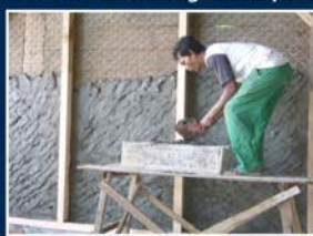
Install backing boards and plaster
